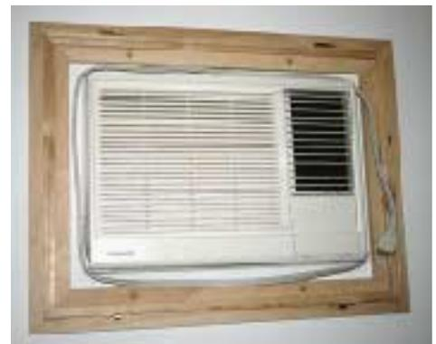
**Figure 5.** Custom-made insulated plywood covers seal attic hatches (left) and through-wall AC units. Cam-type latches and compressible gaskets ensure a tight seal.
