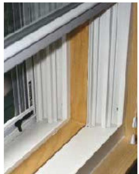
**Figure 10.** Even the windows get doubled in a sound-insulated room. Thermopane glass, minimum 2-inch air spaces between units, and a high-performance storm window present an effective barrier to external noise.
