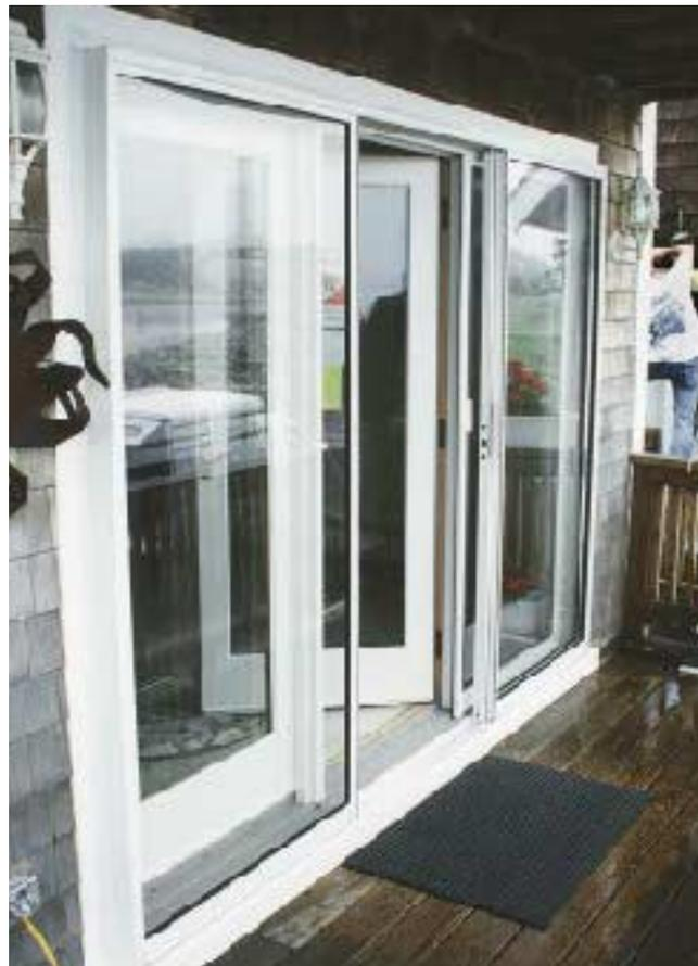
**Figure 3.** Sliding storm panels provide extra sound insulation at sliding door locations. In every instance of a secondary door or window, there should be a minimum 2-inch gap between primary and storm units.
