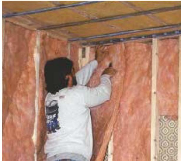
**Figure 9.** Double-wall 2x4 framing set in acoustical sealant caps the top and bottom of an existing boxed-out lower wall section. Fiberglass batt insulation absorbs sound energy. Resilient channel crosses 1x3 strapping over the existing ceiling, which is covered with semi-rigid acoustical fiberglass insulation, followed by a layer of 5/8-inch-thick blueboard with a plaster skim coat.
