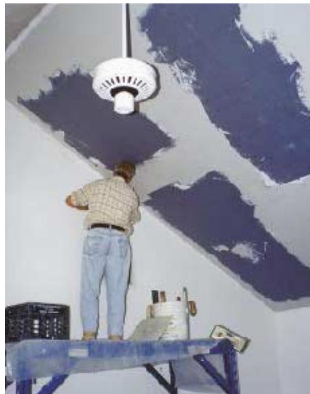
**Figure 7.** Applying the principle that surface mass absorbs noise energy, adding an extra 5/8-inch-thick layer of gypsum blue-board with a plaster skim coat helps to reduce the noise transmitted through flat-roof and cathedral-style ceilings.
