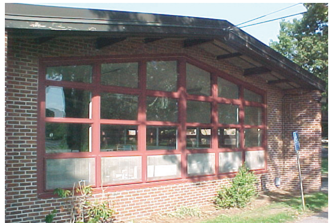
Francis Elementary School
